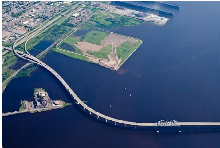
Image courtesy of the Duluth Seaway Port Authority. Photo by Dave Witt/Aero-Environmental Consulting.
